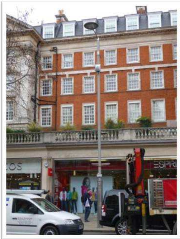
Figure 1 - Rukus 8800 installed in Kensington High Street
